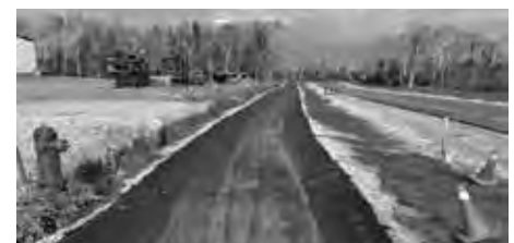
Paved Path at Community Campus
